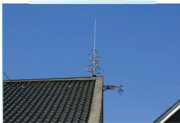
Figure 1.62 (a) Schematic diagram of a lightning arrester. (b) A house with a lightning arrester
